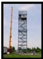
Microwave and Optical Communication Range
